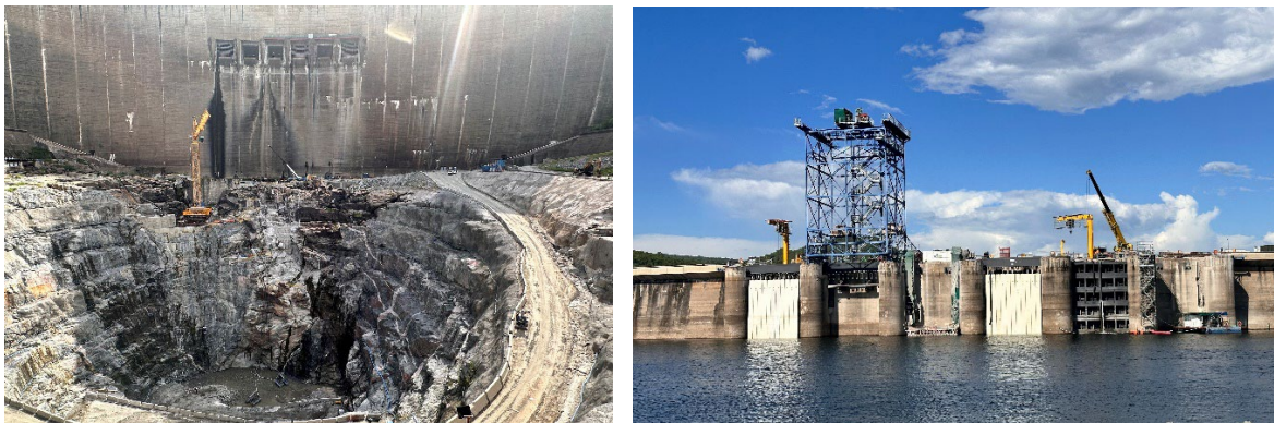
Figure 3 View of the Plunge Pool and Spillway as of December 2023
