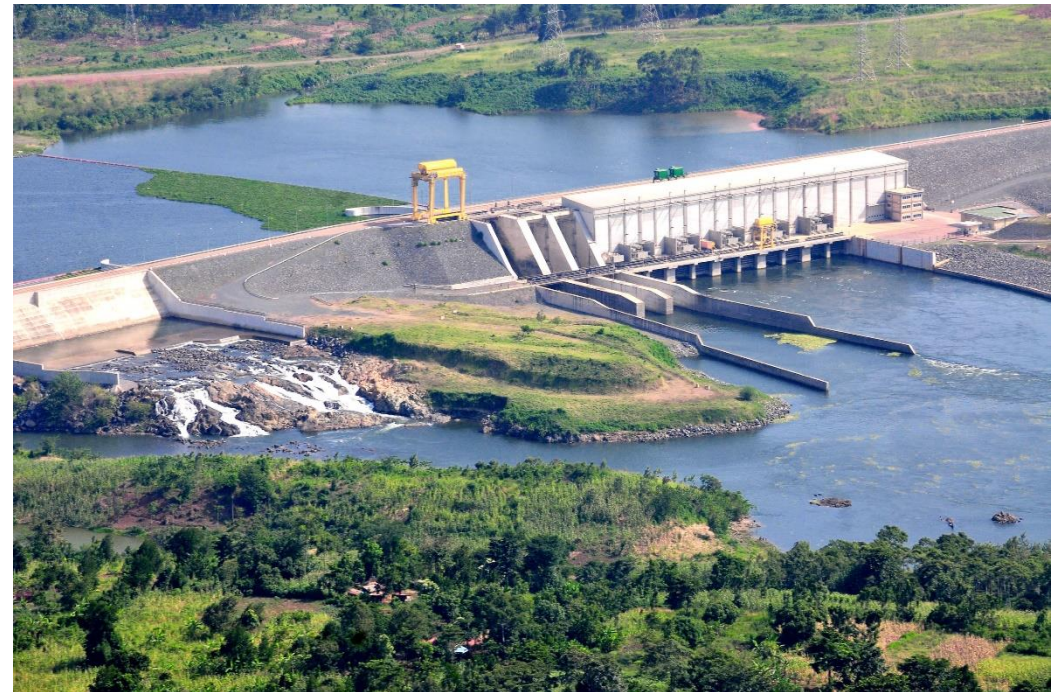
Bujagali HP dam, Eastern Uganda
