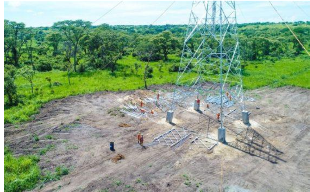
Transmission pylon within Wildlife Reserve
