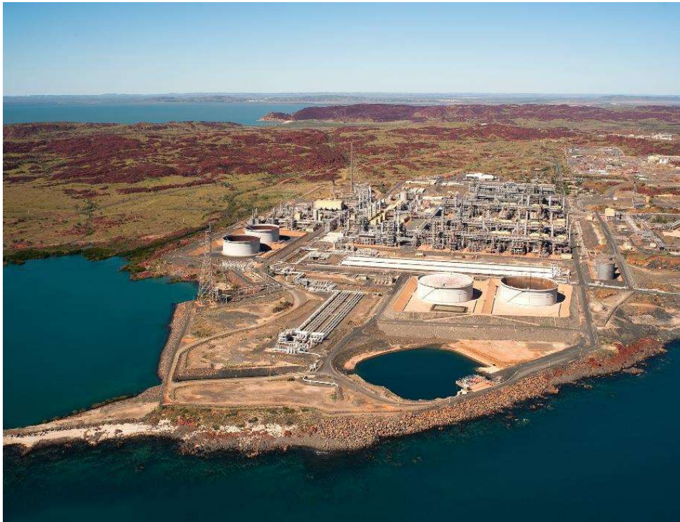
North West Shelf's Project's Karratha Gas Plant
